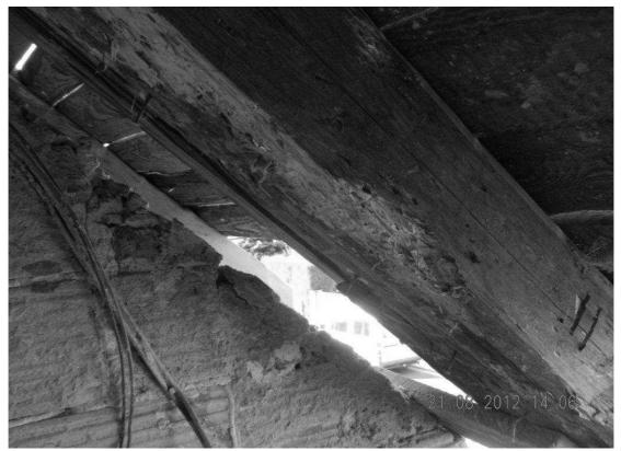
Figura 3 - Photograph of an example of wood-destroying insect action
