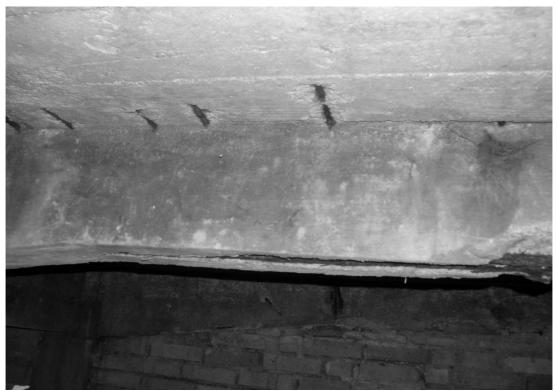
Figura 4 - Photograph of degradation of a reinforced concrete armature.
