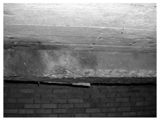
Figure 4 - damage to the reinforced concrete beam and slab
